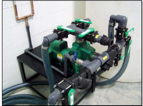
High volume, heavy duty PlantStar /FlowMax pump insures through agitation and quick transfer of materials
