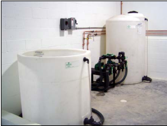
360 gallon open top mix tank with jet agitation and 550 gallon storage tank for rinsate or second mix
